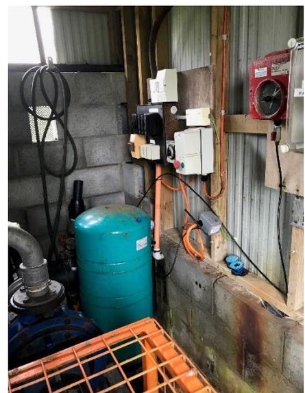
our golf course is watered, whether it be a tee bed, a green, the fairways or the practice green. The jacking pump also operates the sprinklers on the dams which are a nice feature. The bore pump is simply an additional pump to supply water from underground into one of our dams to help with our supply. The bore pump is approximately 30 meters underground and it is under the little silver cover near the pump shed.
